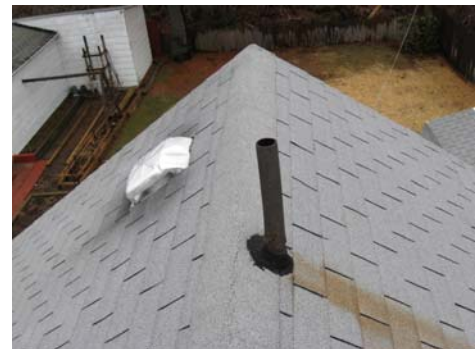
Tar covered flashing at vent
