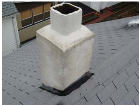
Tar covered flashing at chimney
